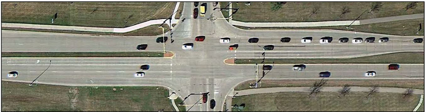
Figure 2-24: Negative Offset Turn Lanes at 32nd Avenue South/ US 81B and 38th Street
